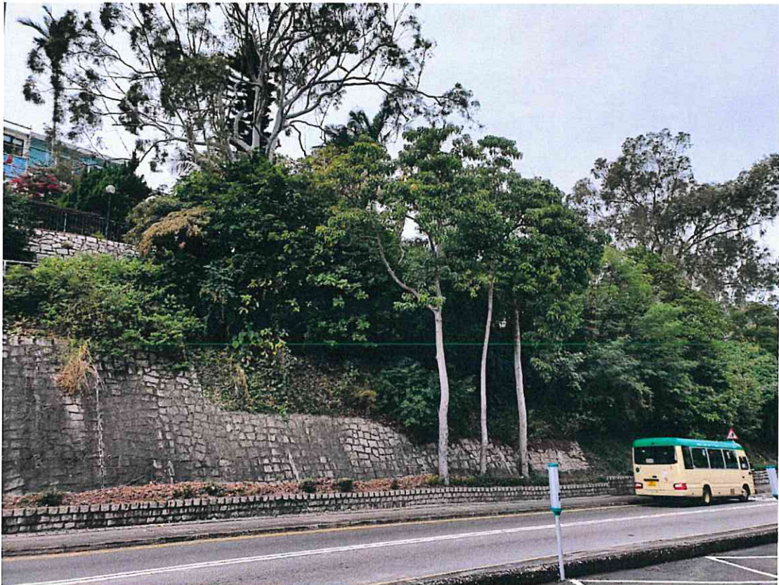
Photo 2: Photo showing the mid portion of Feature No. 7SE-D/C86
