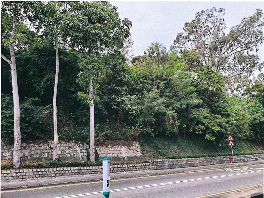
Photo 3: Photo showing the northern portion of Feature No. 7SE-D/C86
